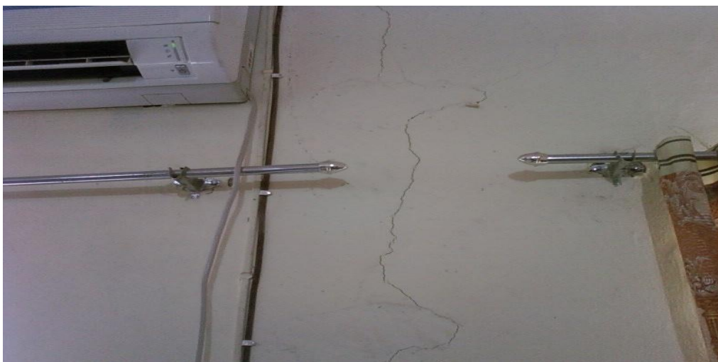
Plate 15 Acceptable Cracks.
