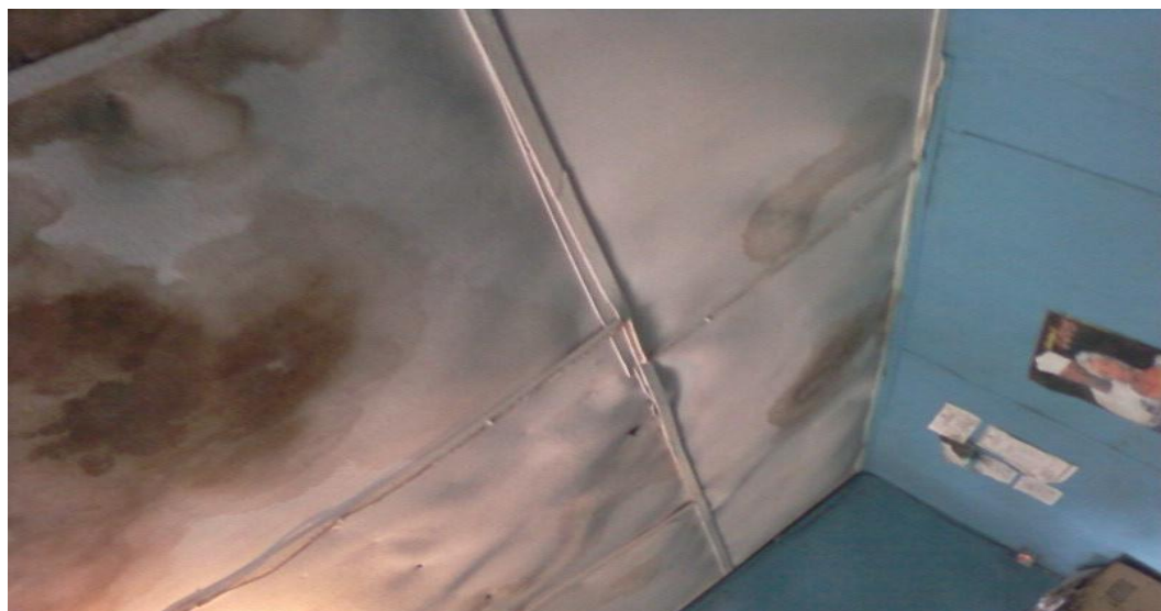
Plate 4 Roof defect
